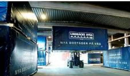
5. Storage of volume modules
