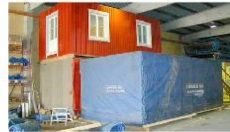
4. Exterior completion and covering
