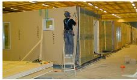
2. Assembly to volume modules
