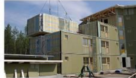
7. Erection of modules on site
